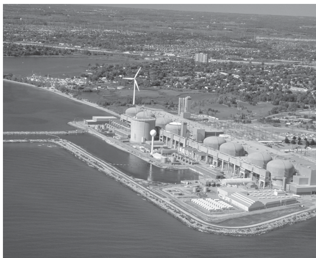
The Pickering nuclear generating station is focusing on plant life maintenance and life extension.
