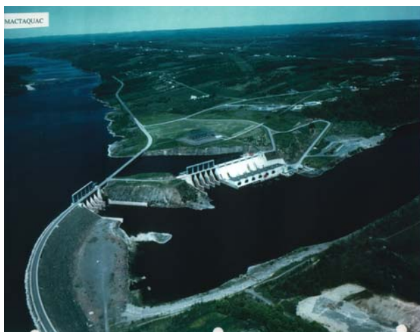
Mactaquac Hydro Station (660 MW)
